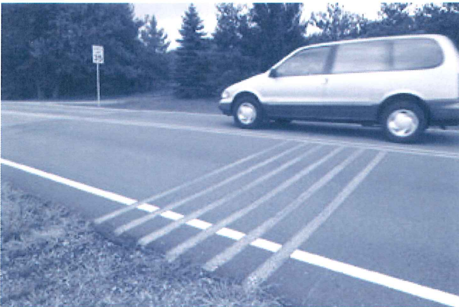
Picture No. 4 Transverse Rumble Strips
