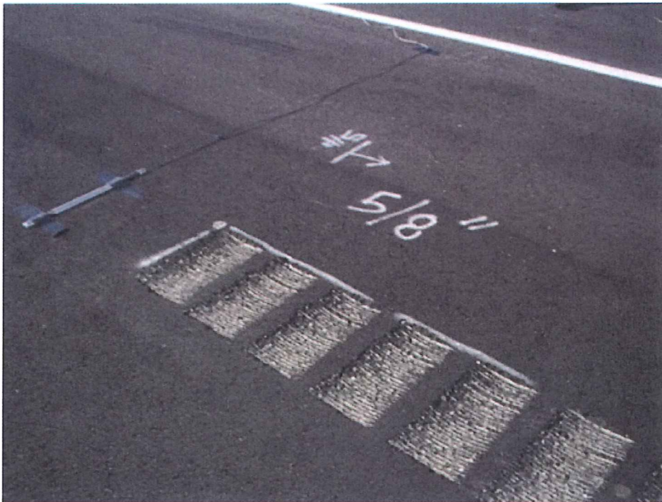
Picture No. 3 Rumble Strips
